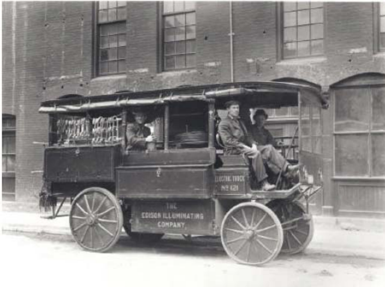
Edison Illuminating Company electric overhead line truck, 1915
