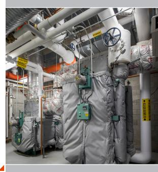
The heat exchangers transfer the exhaust heat from the micro turbines to generate hot water.
