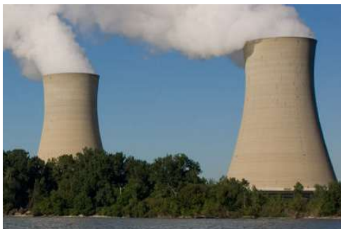
FERMI 2 NUCLEAR PLANT
