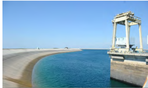
LUDINGTON PUMPED STORAGE
