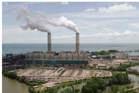
MONROE POWER PLANT
