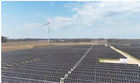
PINE RIVER SOLAR AND WIND PARK
