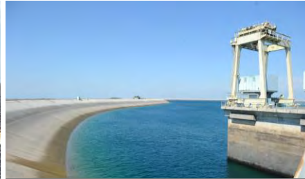
LUDINGTON PUMPED STORAGE
