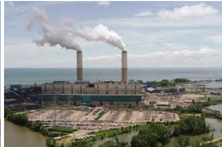
MONROE POWER PLANT
