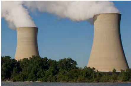
FERMI 2 NUCLEAR PLANT
