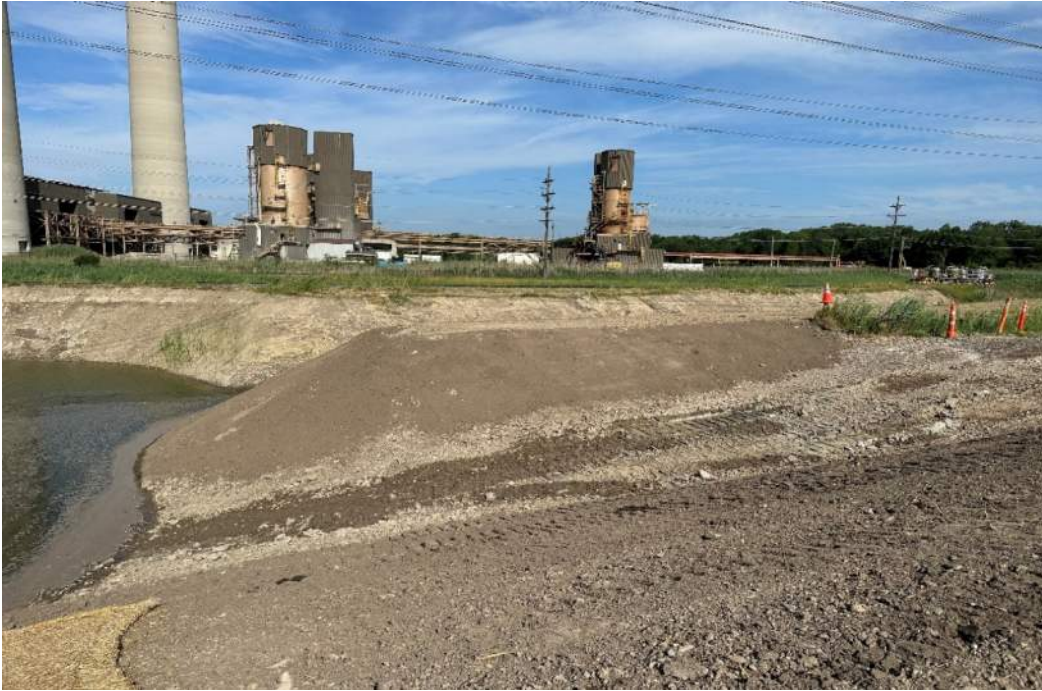
Photo 16: Ramp area, CCR removal and overexcavation complete, Looking W. (7/11/2023)
