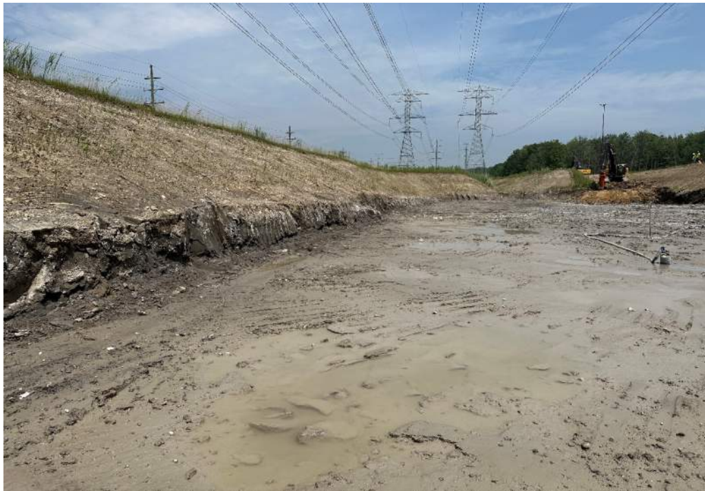
Photo 11: Excavation at west slope, looking north (6/29/2023)
