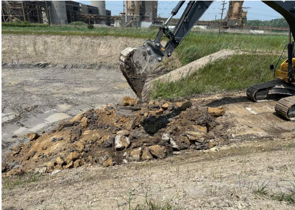
Photo 12: Removal of hardened CCR and overexcavation, in the ramp area (6/29/2023)
