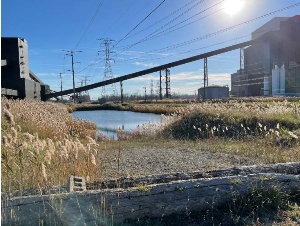
Photo 2: Diversion Basin pre-construction, access ramp looking S. (11/07/22)
