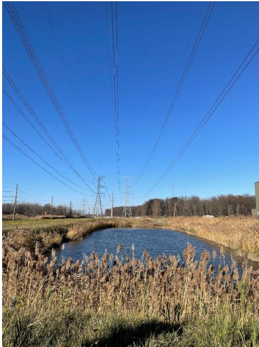
Photo 1: Diversion Basin pre-construction, S end looking N. (11/07/22)
