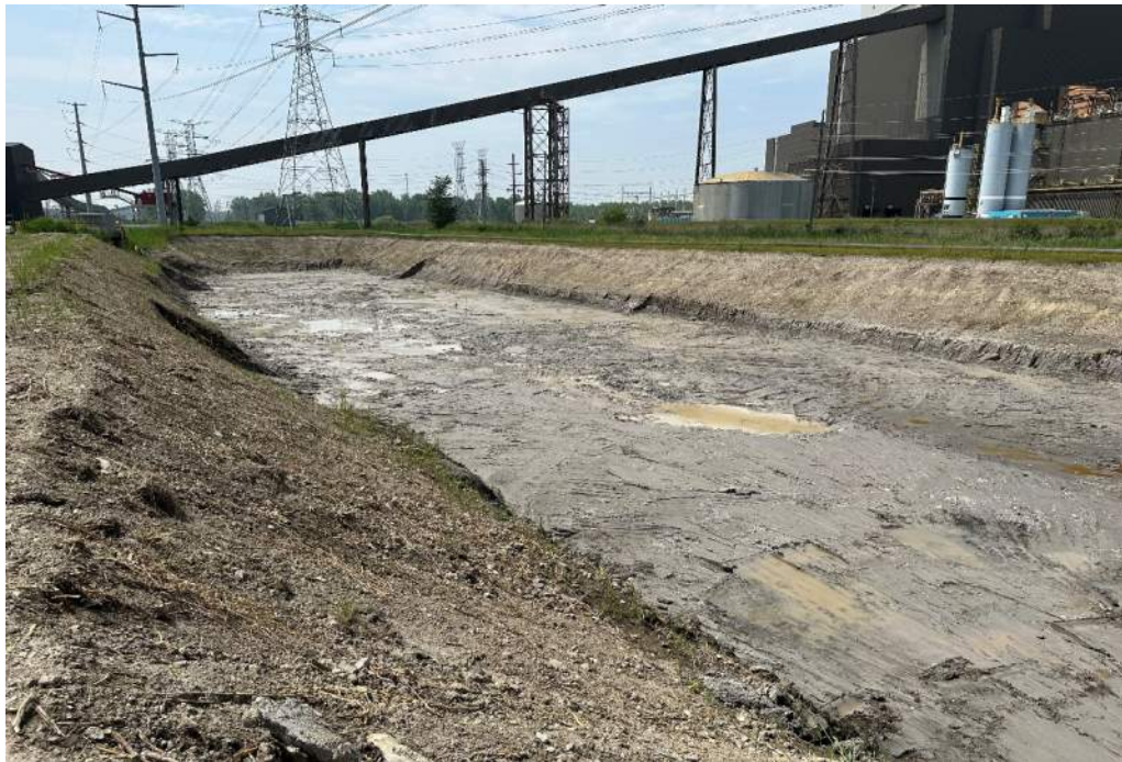
Photo 9: Overview of completed CCR removal and overexcavation in Diversion Basin (6/29/2023)
