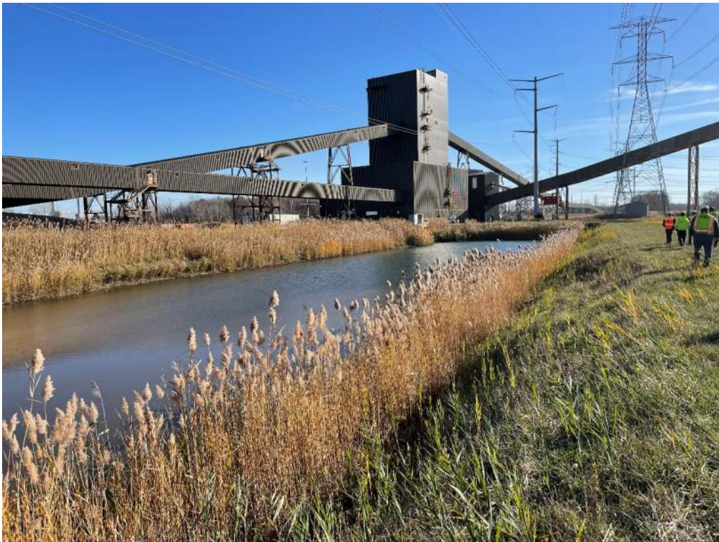
Photo 5: Diversion Basin pre-construction, W slope looking SE. (11/07/22)
