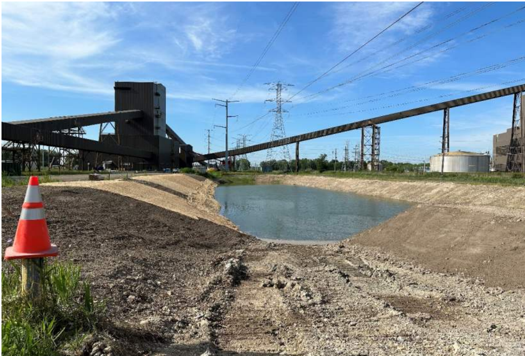
Photo 17: Ramp area, CCR removal and overexcavation complete, Looking S. (7/11/2023)
