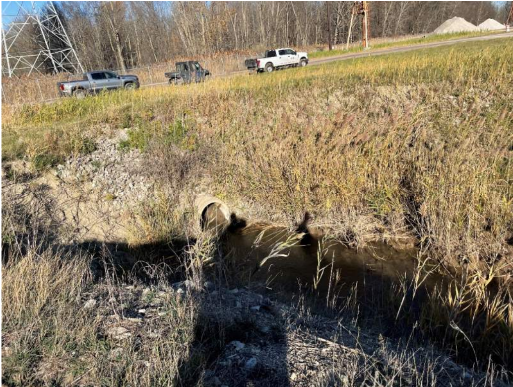
Photo 3: Diversion Basin pre-construction, inlet at N channel. (11/07/22)
