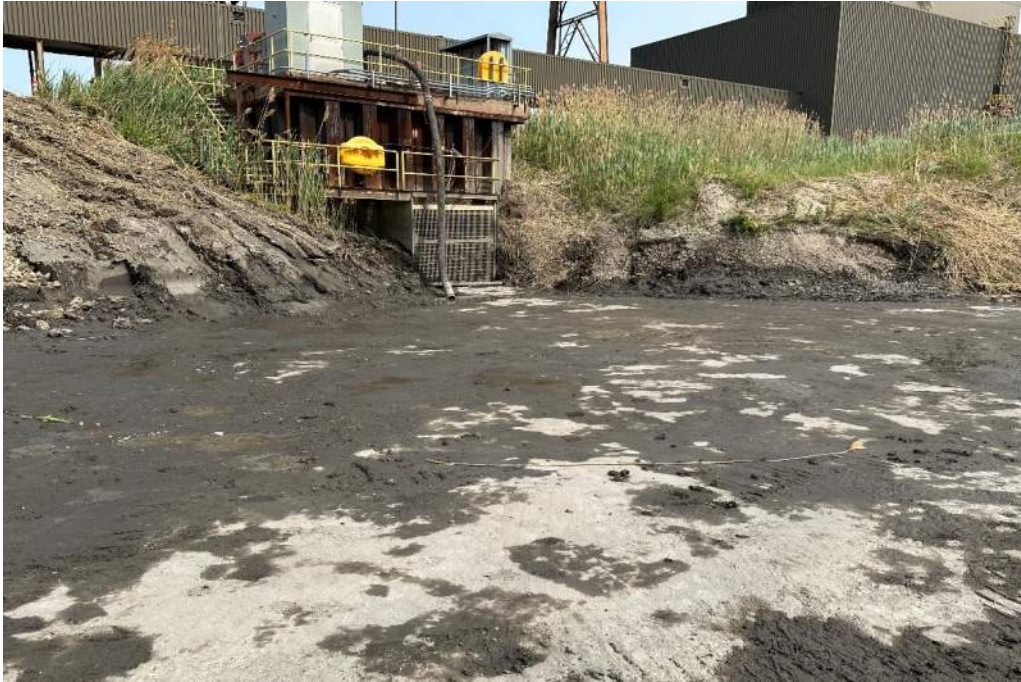
Photo 8: Typical Diversion Basin slopes prior to excavation of hardened CCR material (6/6/2023)
