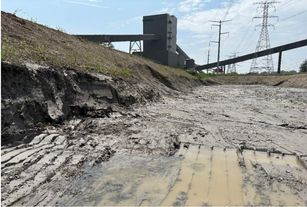
Photo 10: Excavation at east slope, looking south (6/29/2023)
