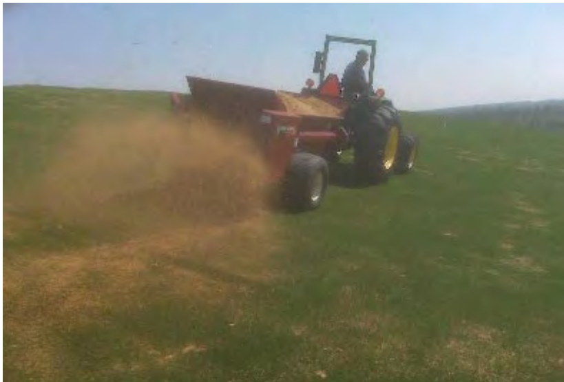
Figure 3-1 Rubber-Tired Construction Equipment on ClosureTurf System
