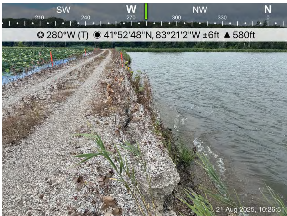
Surficial cracks and sloughing along separation berm
