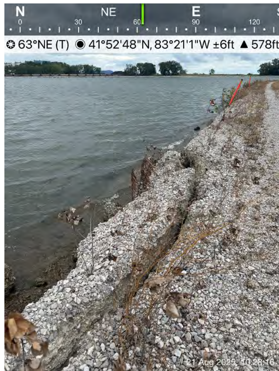
Surficial cracks and sloughing along separation berm
