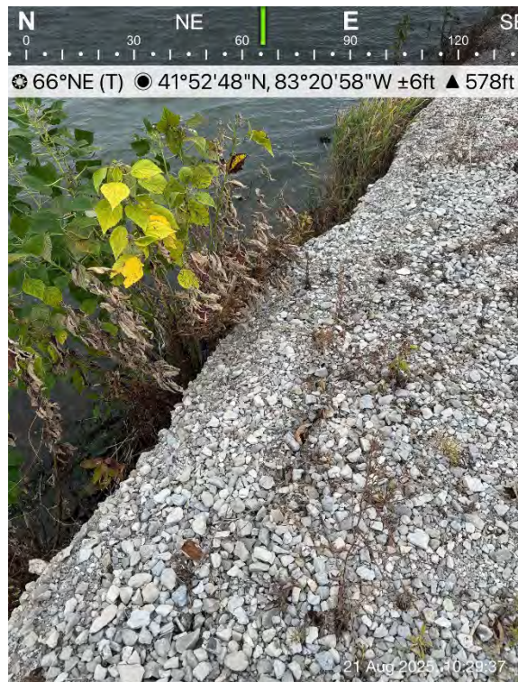
Surficial cracks and sloughing along separation berm
