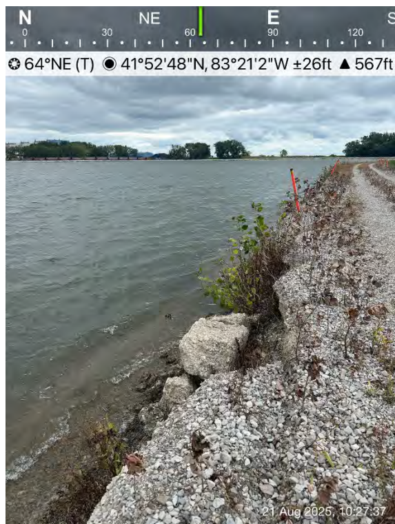
Surficial cracks and sloughing along separation berm
