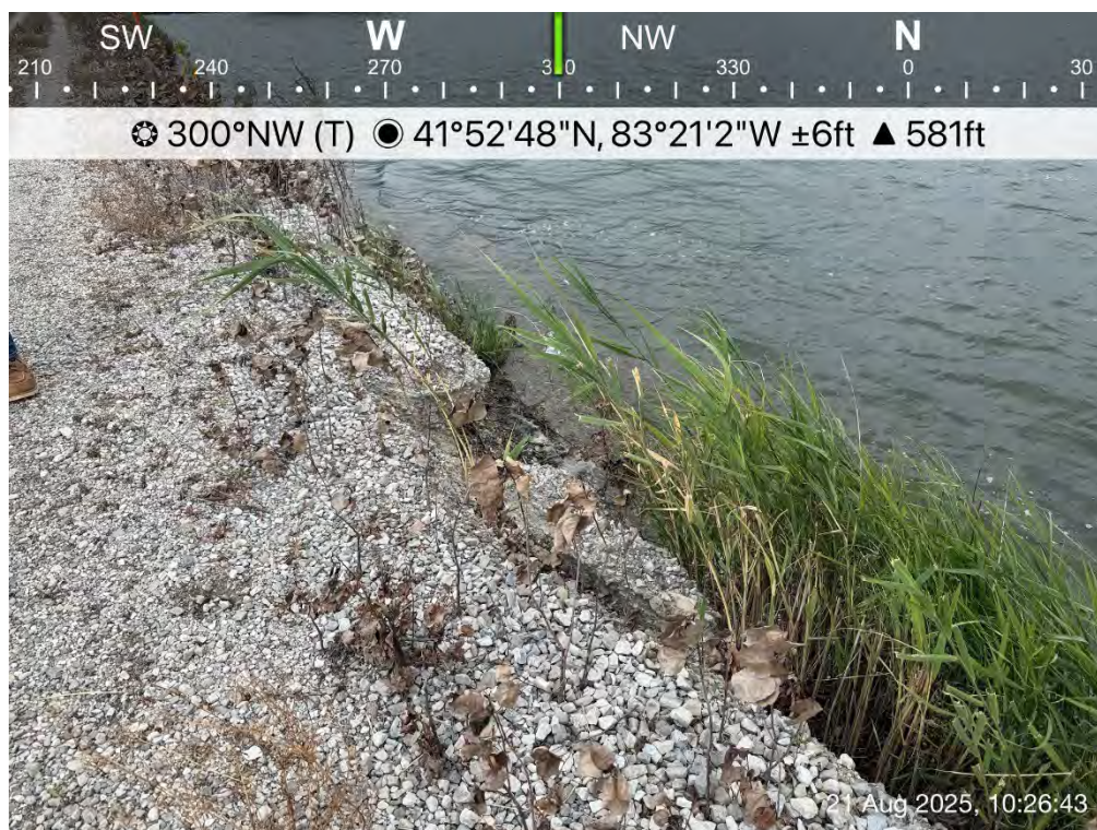
Surficial cracks and sloughing along separation berm
