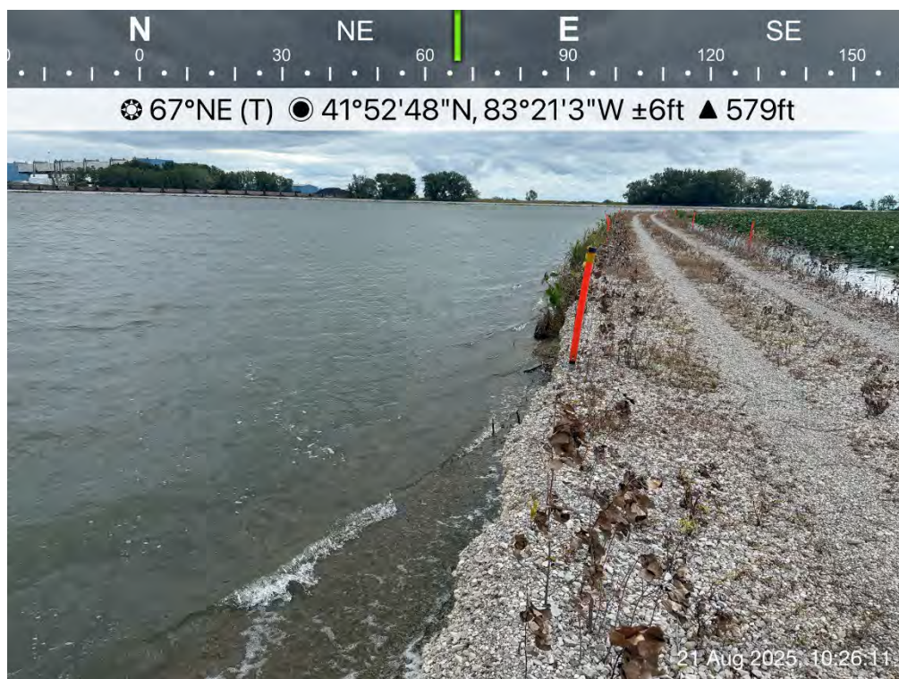
Sloughing along separation berm
