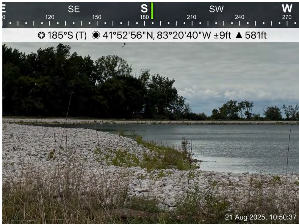
Finished north and eastern closure armoring with vegetation
