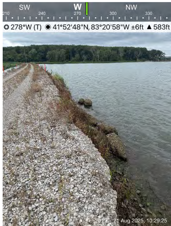
Sloughing along separation berm
