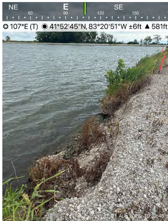
Sloughing along separation berm
