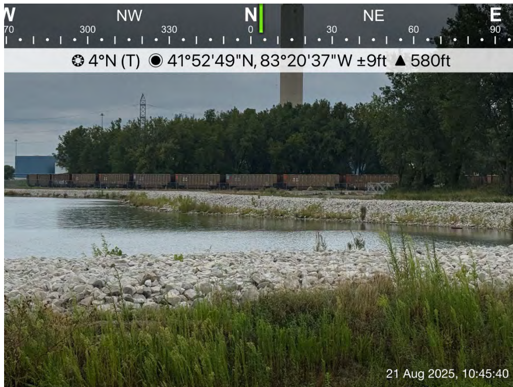
Eastern perimeter of impoundment with finished closure armoring and vegetation
