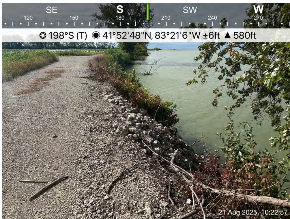
Rip-rap armoring along western exterior embankment
