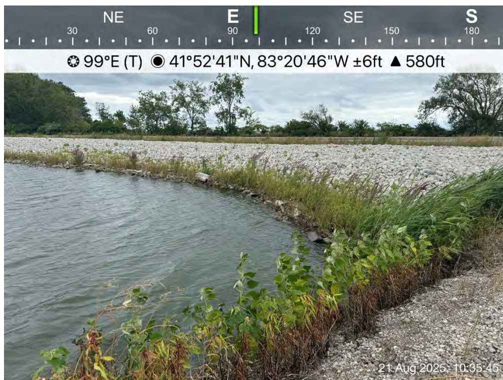
Southeast corner of impoundment with finished closure armoring and vegetation
