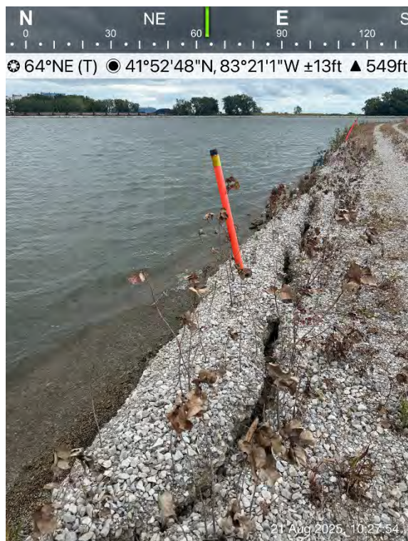
Surficial cracks and sloughing along separation berm
