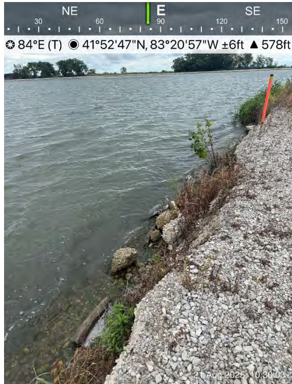
Sloughing along separation berm
