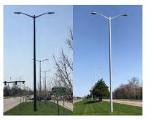
DTE Post Code 71/73 & 81/83: 30' or 40' black or silver dual arm fiberglass direct bury post with breakaway base.
